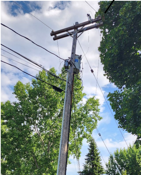
Circuit #3-6 Prospect Street Tight Clearances
