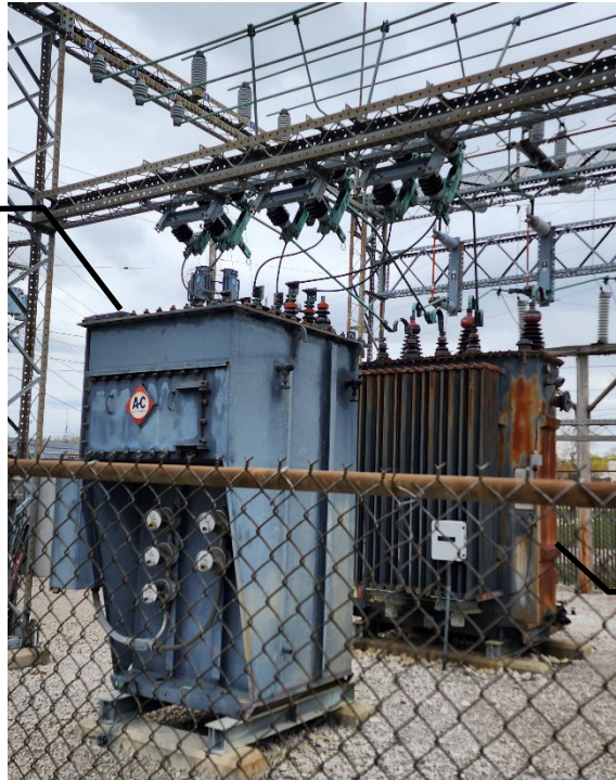
2400V Transformer & Voltage Regulator Consumer Energy Owned Equipment
