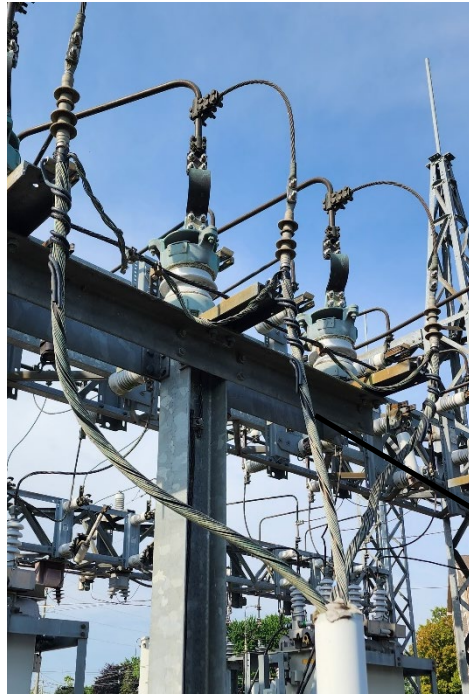
4.16kV Substation Circuit Exit Aged Underground Cable
