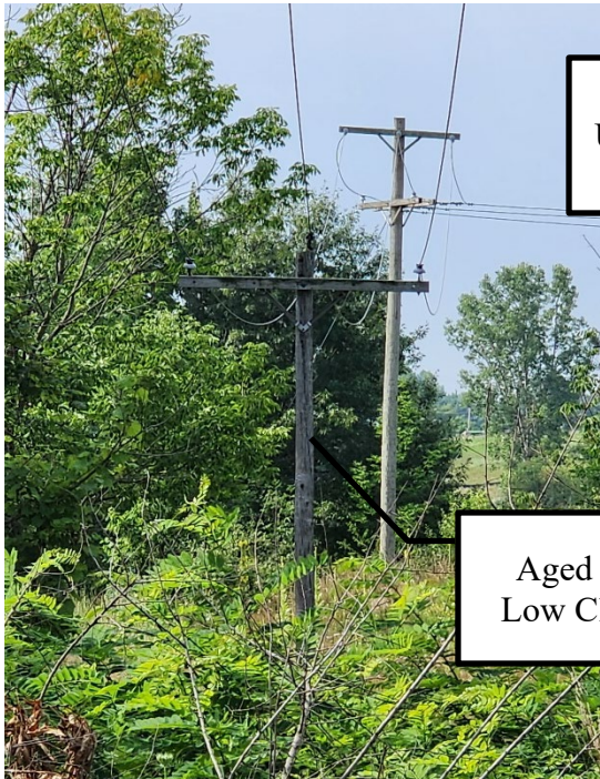
Circuit #3-6 Prospect Street Aged Construction & Low Clearance
