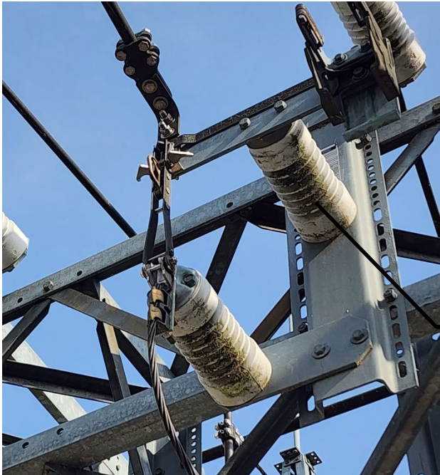
4.16kV Substation Contaminated Insulators
