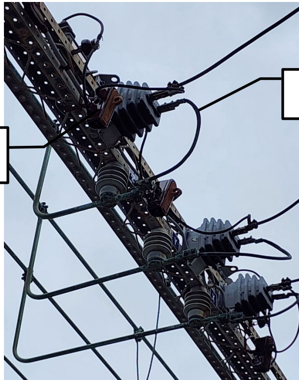
4.16kV Substation Metering
