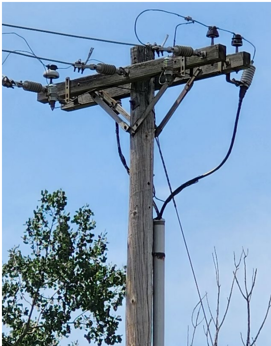
Evergreen Village Unjacketed Concentric Neutral Cable
