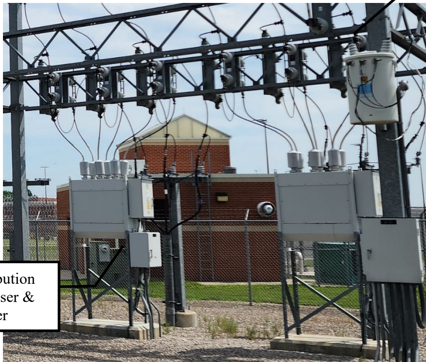
Gibson Substation Distribution Circuit Reclosers
