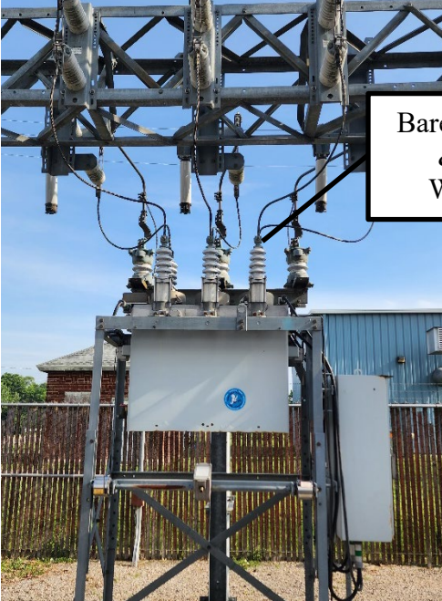
4.16kV Substation Distribution Circuit Recloser
